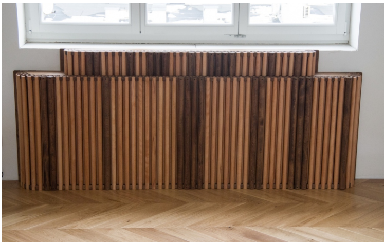
The radiator cover. Made of oak and beech wood, covered with a mixture of wood stains and tung oil.
